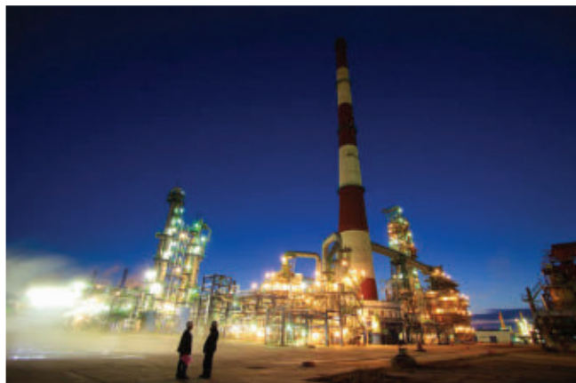
JSC Gazprom Neft has let a contract to RusTechnip for a CDU-AVT complex at its 21.4 million-tpy Omsk refinery in Western Siberia. Photo from Gazprom Neft.
